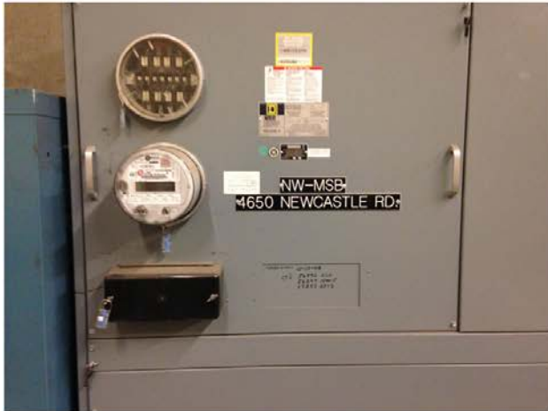
FIGURE 11: VIEW OF MSB METER SECTION
